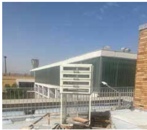
Building Ventilation using solar chimney new design in students' graduation project
