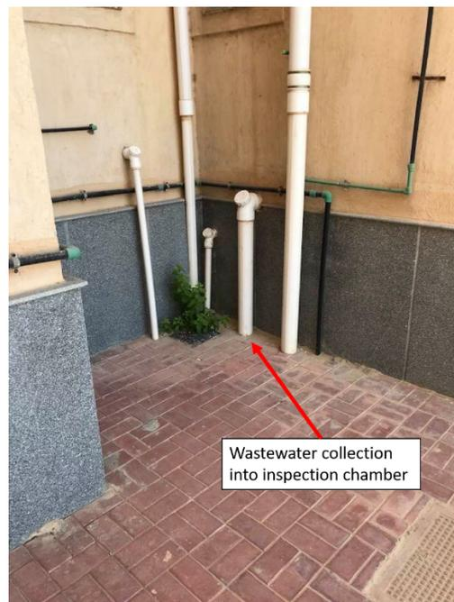
Collection of wastewaters (separate pipes of grey and black water) from each flat
