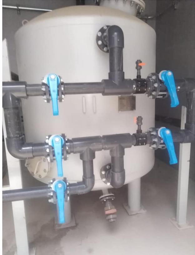
Sand filtration system to treat portion of wastewater (120 m<sup>3</sup>/d) at EJUST
