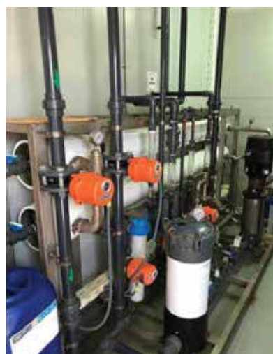
Reverse osmosis desalination unit at E-JUST campus, providing safe and free drinking water
