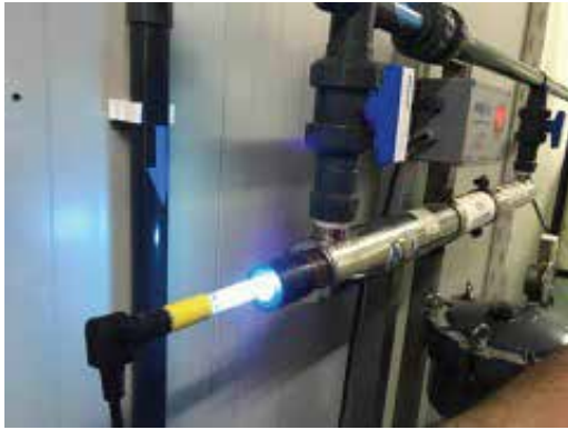
Ultraviolet (UV) unit for disinfection
