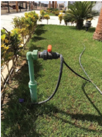
Drip irrigation system to minimize water loss
