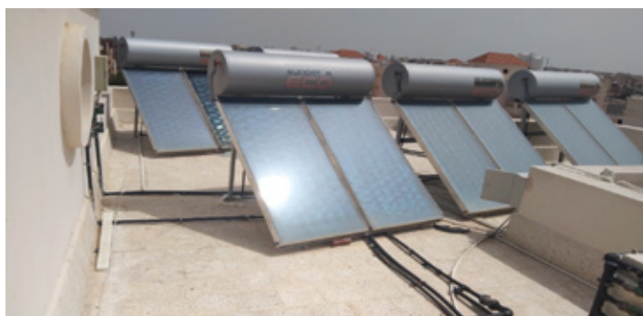
Solar water heating in housing buildings
